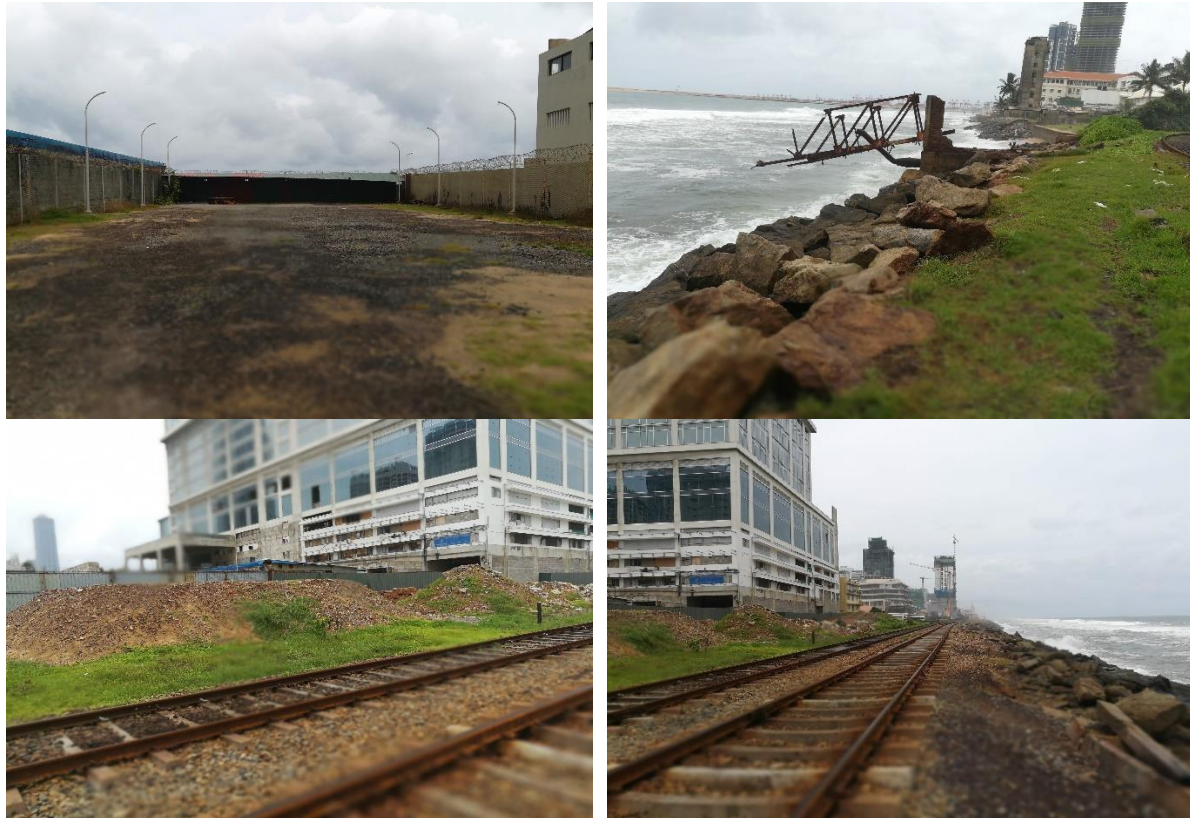
Figure 02-13 Existing condition of the project site
