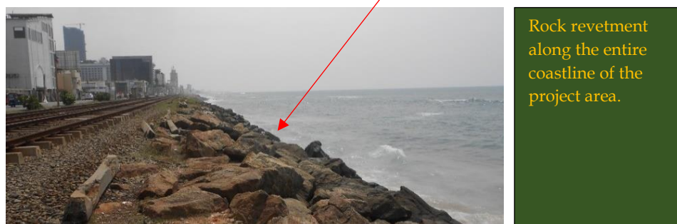
Figure 03-10 Revetment at the front of the proposed development project.
